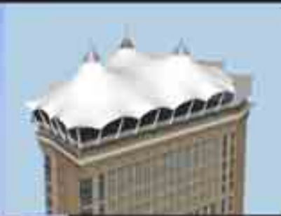
wind loads on light weight structures
